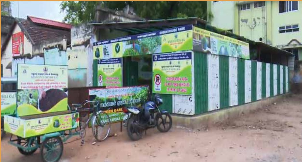
Composting Unit at the Public Parking lot
