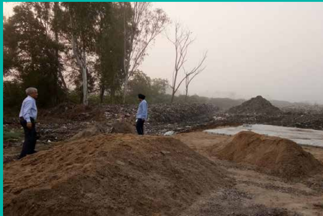
Remediation of the existing dumpsite
