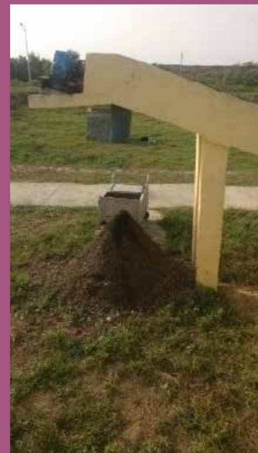
Sand extracted from the grid chamber
