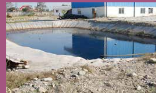
Solar Evaporation Pond
