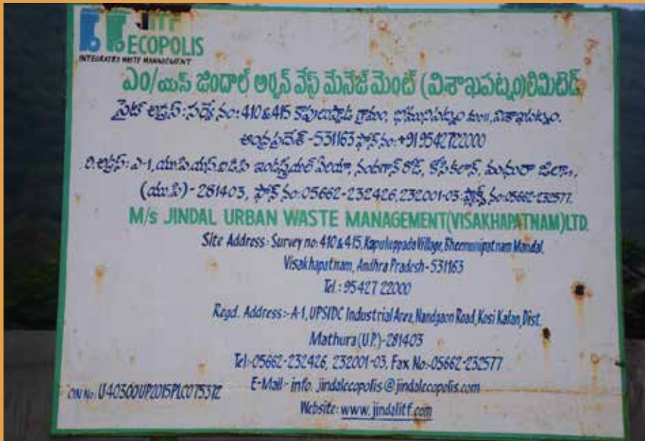
WTE Plant under construction
