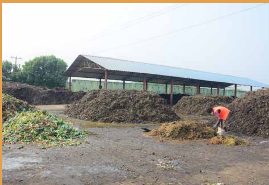
Gajuwaka Windrow Composting Unit
