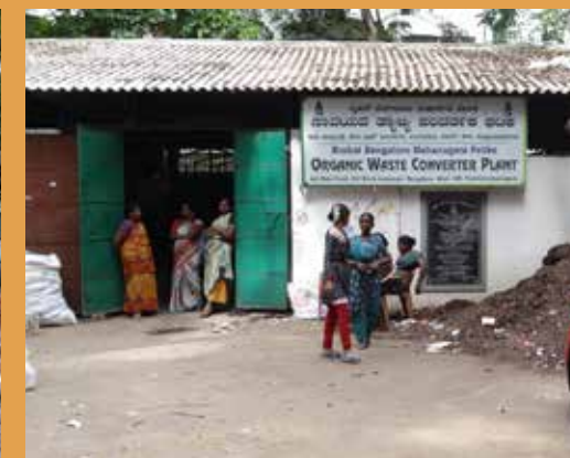
Organic Waste Converter Plant
