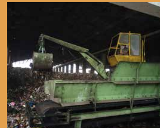
Mechanical composting plant at Moshi
