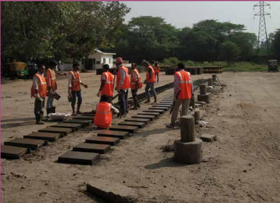
Concrete mix is poured into the frames and left to set
