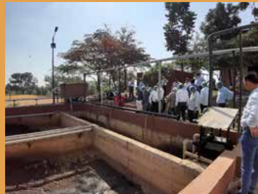
Leachate treatment plant
