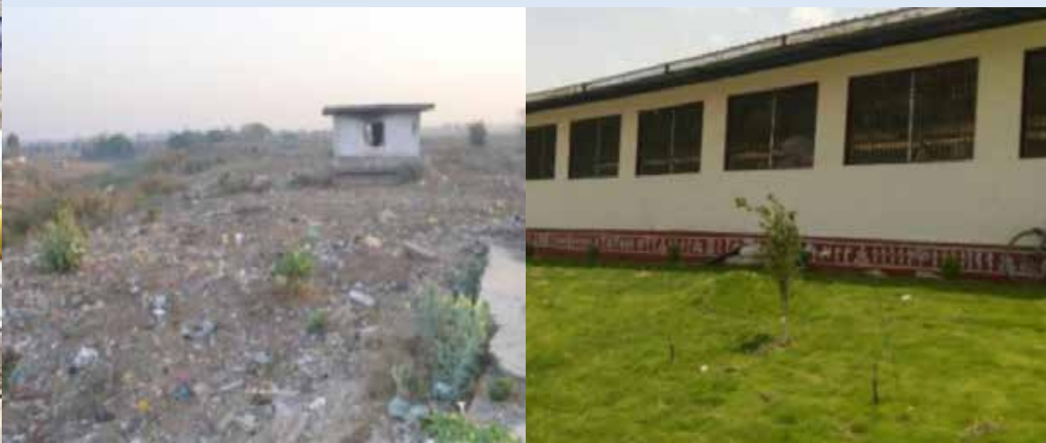
Conversion of Dumpsite to Sanitary Park
