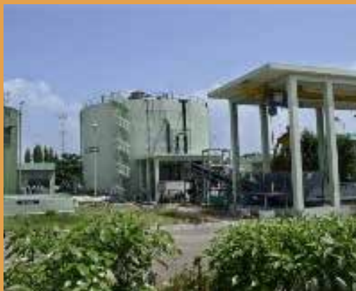
Biomethanation Plant for Power Generation in Koyambedu Vegetable Market
