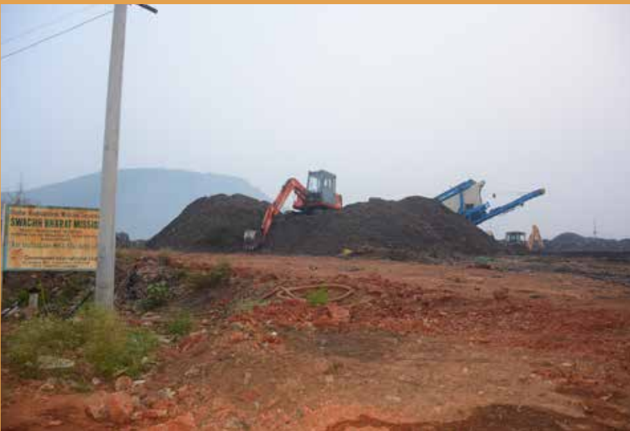
Biomining process being carried out at Kapuluppada Landfill Site
