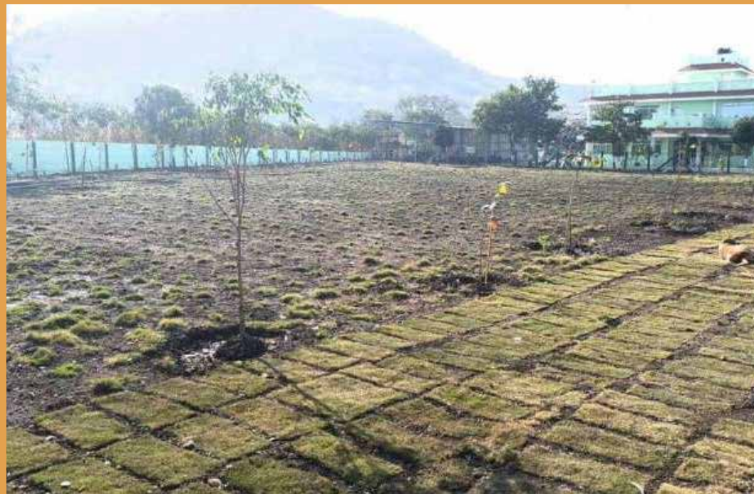
Centralized Organic Wet Waste Processing Unit
