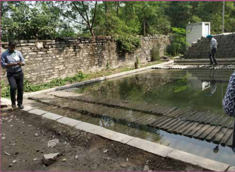
The Concrete tiles are put in pond for curing
