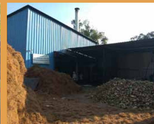
Coconut Waste Processing Unit
