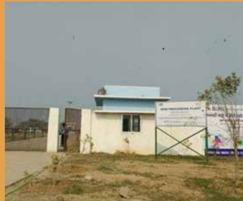
Composting Plant at Karsada
