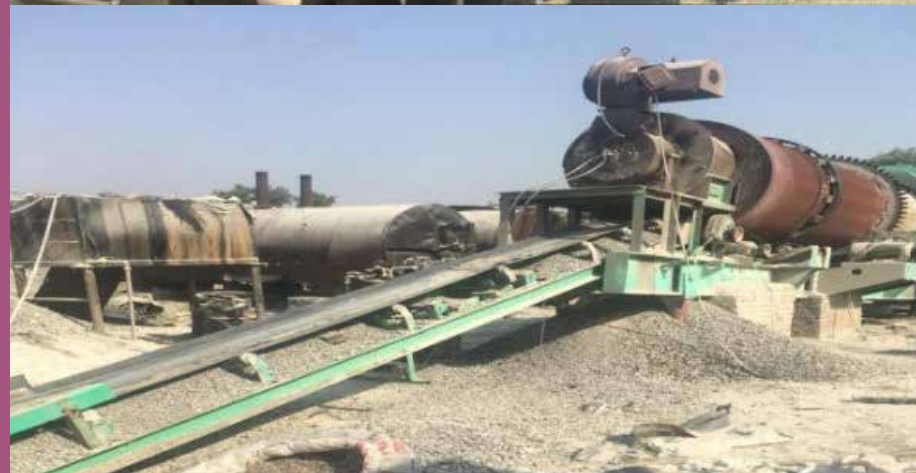
Use of Plastic Waste in road making
