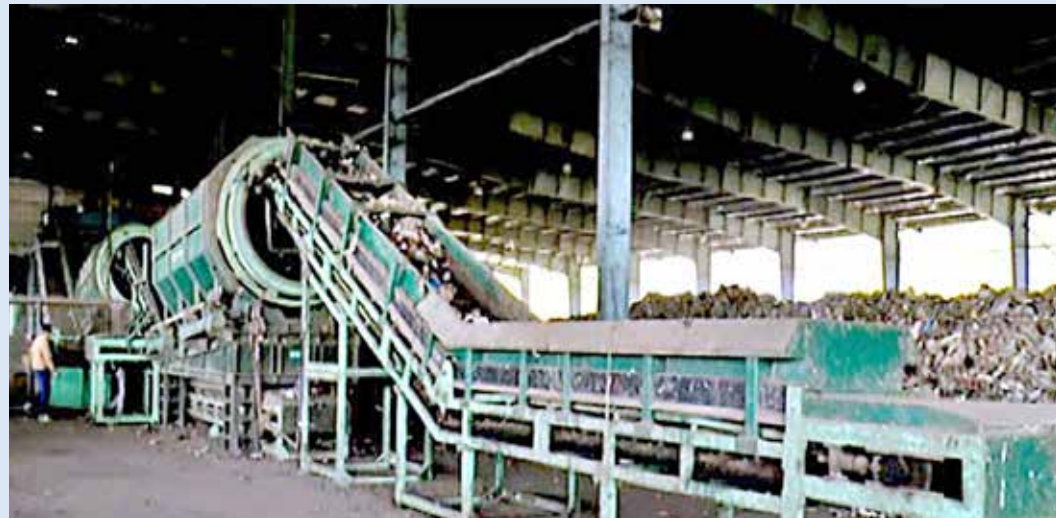
Solid Waste Treatment Plant, Lamdeng
