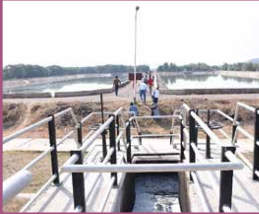
Waste water transferred to the Anaerobic and Facultative ponds
