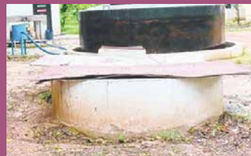
Biogas Plant at XLRI
